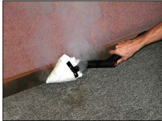
Steam cleaning the baseboard. Note that the wand is covered with a terry wash cloth to increase and retain heat. Photo by R. Cooper.
