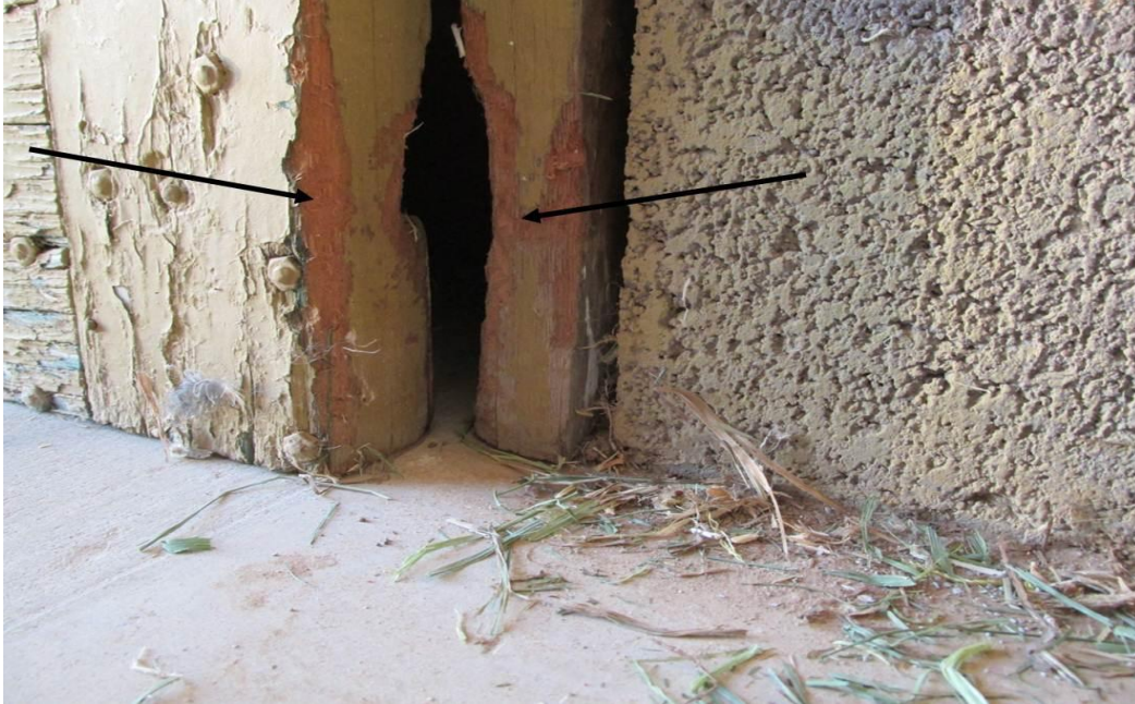
Figure 19: Evidence of packrat gnawing activity. Figure credit: Charles Conner.
