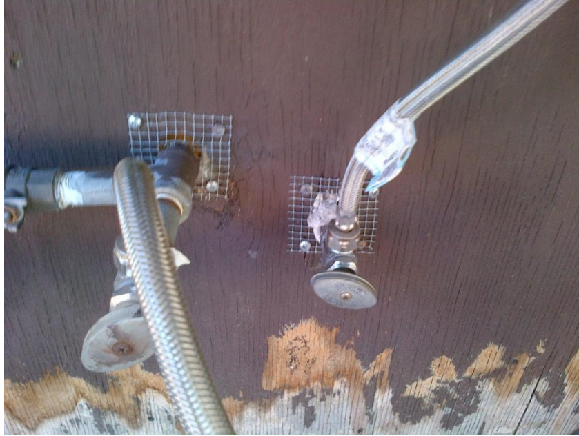
Figure 29: Methods to fill gaps can include caulk and ¼ inch hardware cloth fastened with a staple gun or screws. Figure credit: NPS Figure.
