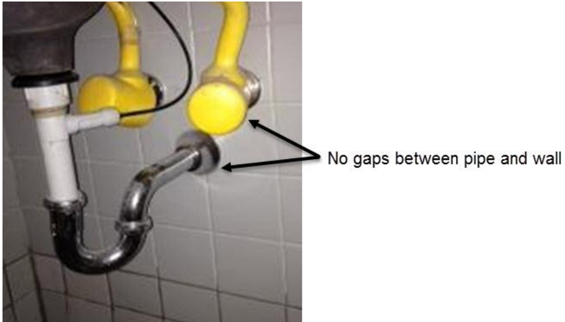
Figure 16: Evaluate service entry points. Here plumbing entrance points are sealed using a commercial flange that is sealed to the wall tile using caulk. Figure credit: NPS Figure.
