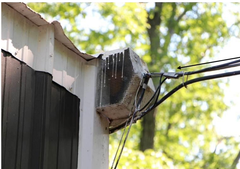
Figure 12: Electrical cables covered with ¼" hardware cloth at the cable/roof junction to exclude rodents at the cable entry point. Figure credit: NPS Figure.
